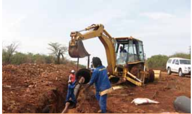
Construction of ductile rising main to Zigagayi 2.5 ML reservoir
