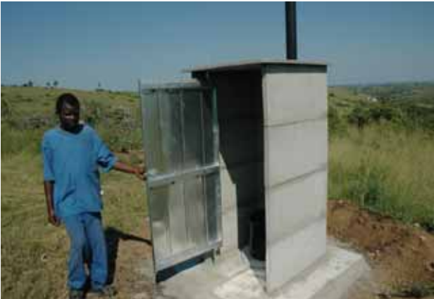
Mbonambi sanitation concrete structure
