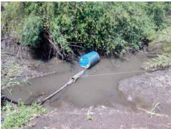
The above photos show the Bangicala River intake, which has dried up and is now being serviced by a water tanker.
