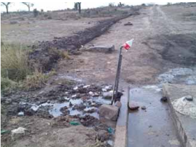
The photo above shows a trough that was excavated next to a communal standpipe by community members for their cattle to have access to water.
