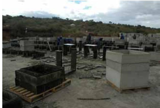
Precast yard production at the uMlalazi Precast yard
